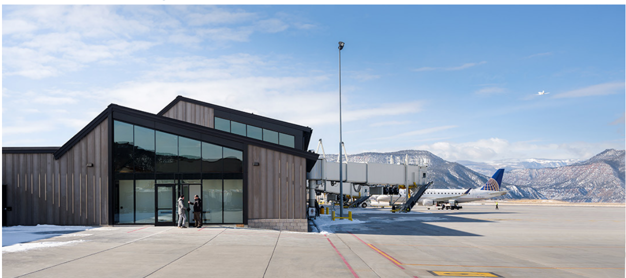
Figure B-7 – Concourse Exterior
