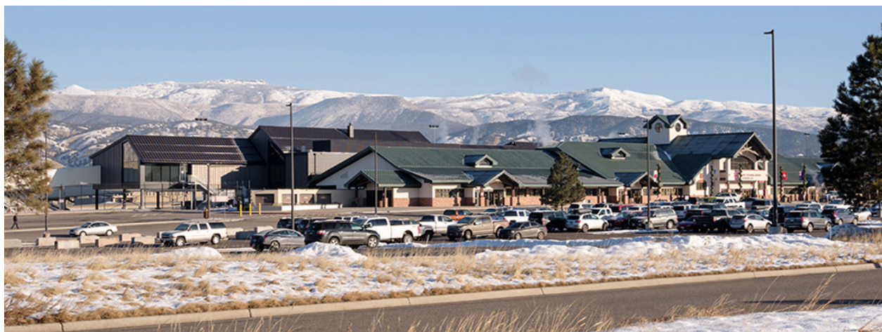
Figure 2-8: Commercial Terminal Building
